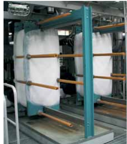
Fig. 5 Due to flexible design, no damage will occur when freezing.
