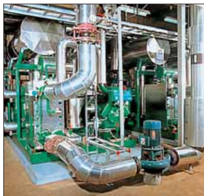
Fig. 2 The AlfaRex TM10-B ammonia evaporator and condenser in a chiller heat pump system with ammonia as refrigerant installed in a Danish research institute. The system was built by Sabroe.
