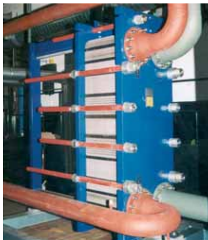
Fig. 2 SWPHE as an evaporator in a brewery installation.
